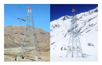
Fig 3. 220 kV S/C Single ACSR Deer T.T. 'D' with cross arm staggering
