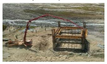
Fig 23. Casting of foundation
