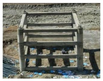
Fig 4. Special Foundation with Circular straight pedestals and tie beams
