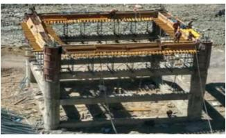
Fig 22. Scaffolding Installation
