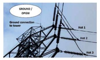
Fig.3 Arrangement of Conductor and Ground wire on Tower
