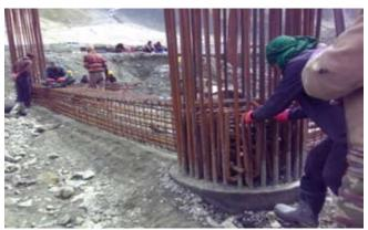
Fig 21. Reinforcement bar tying
