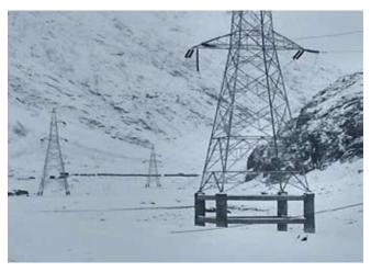
Fig 5. Raised Chimneys for increased clearance for conductors
